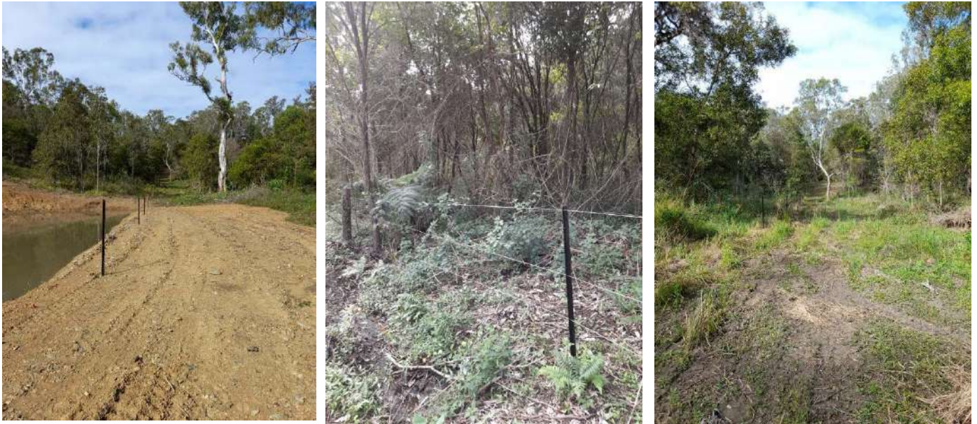
Photo set 1: Fauna friendly fencing installed along cleared boundary.
