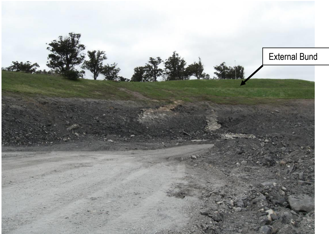
Plate 5 – External Bund Constructed from Overburden
