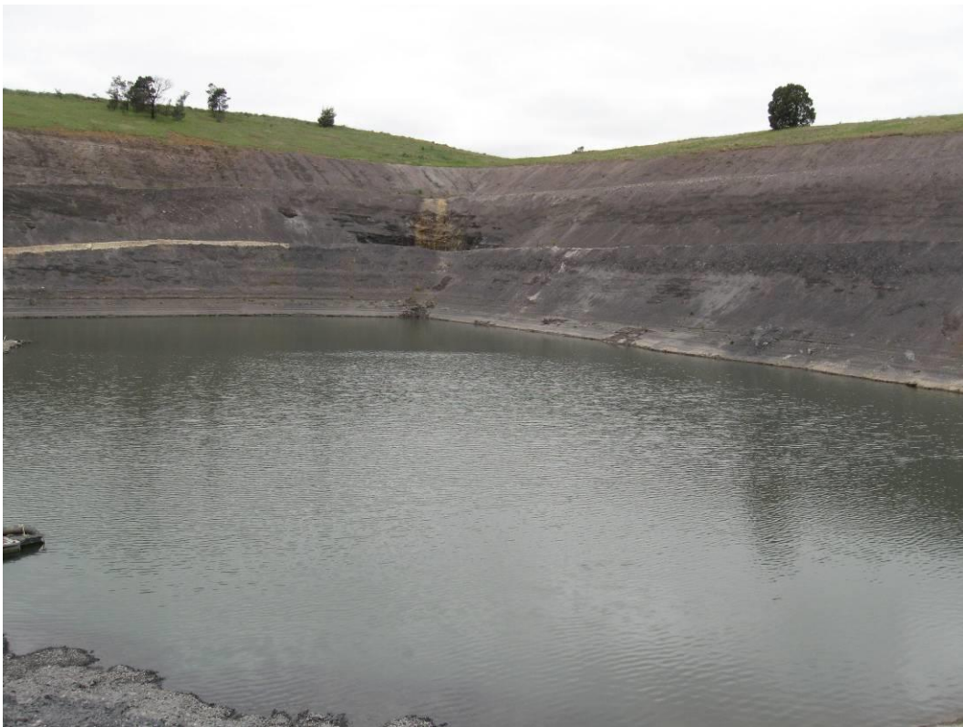
Plate 2 - Water Storage in Eastern Void
