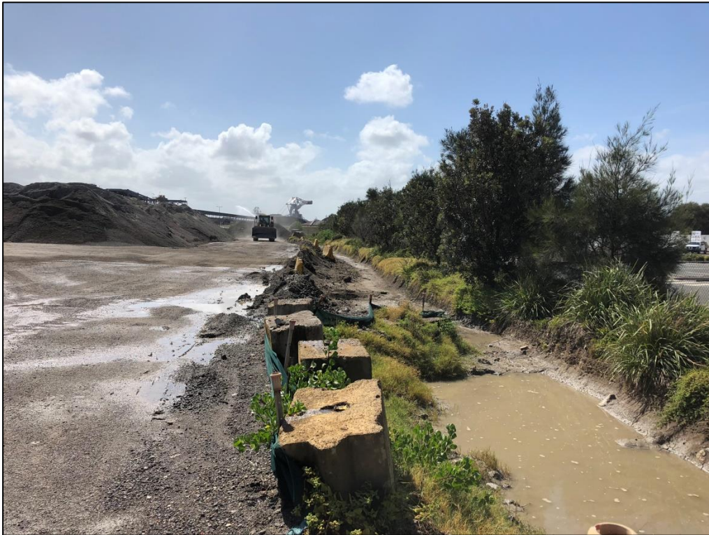
Figure 2: Looking north-west along drainage swale from near the weighbridge.
