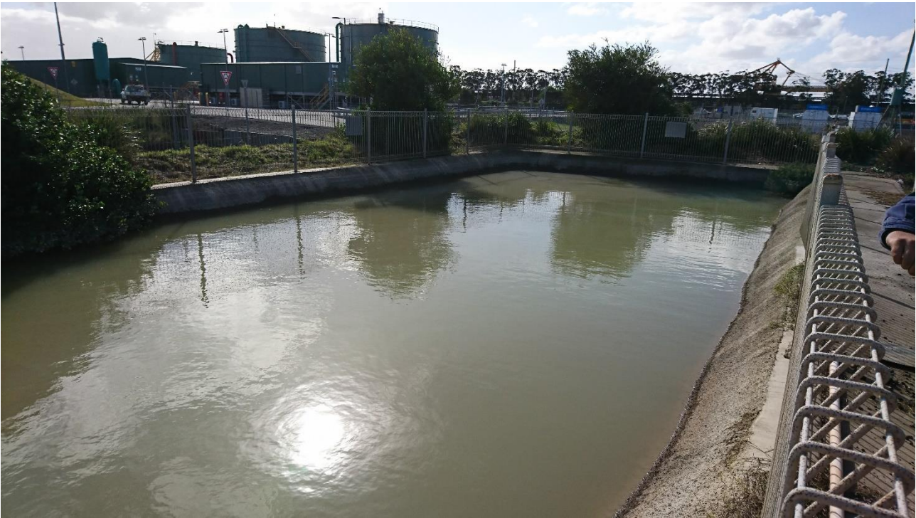
Photograph 2.2 Concrete-lined basin
