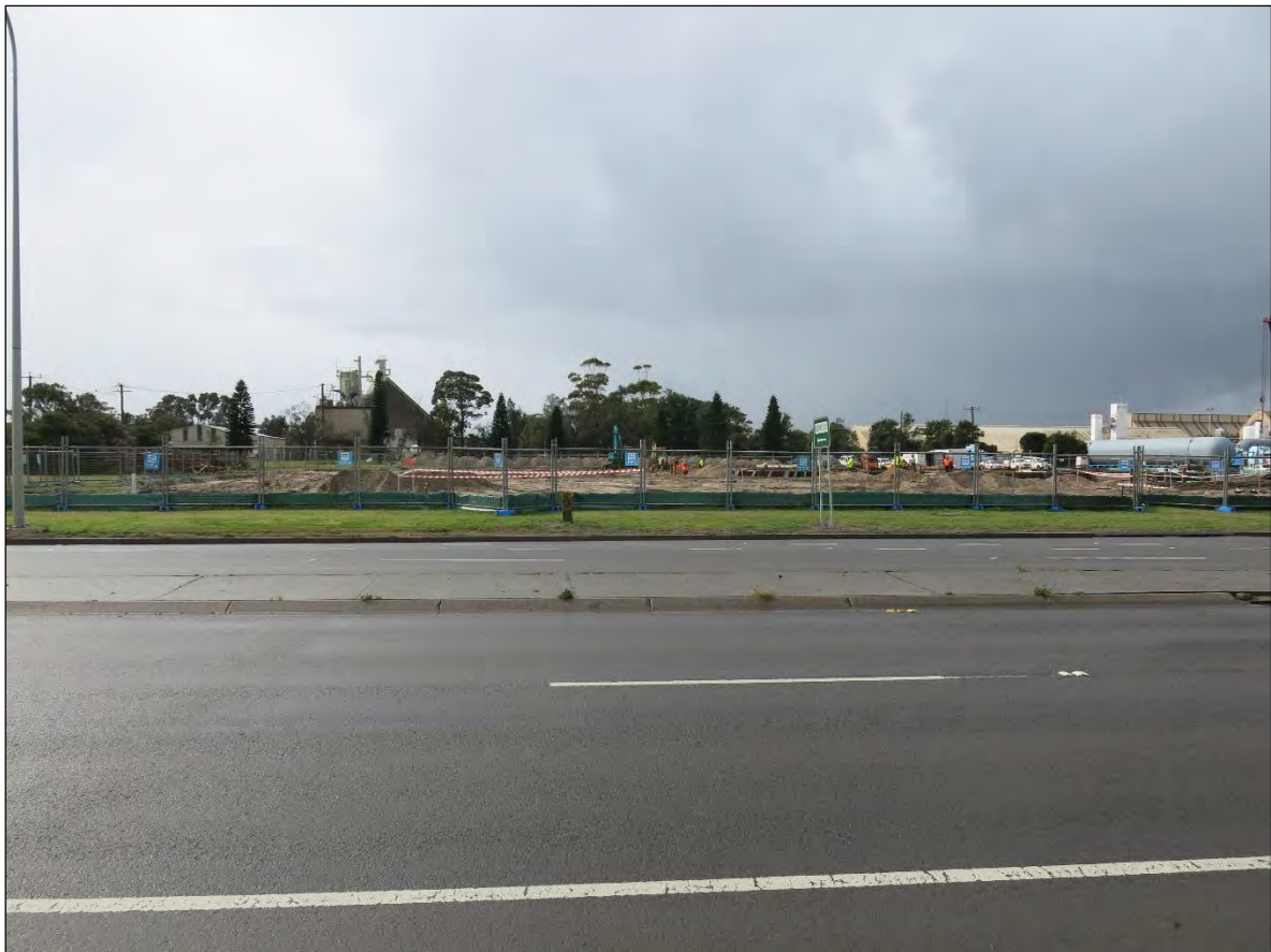
Plate 2 – View from Cormorant Road towards site with service station under construction in middle ground.
