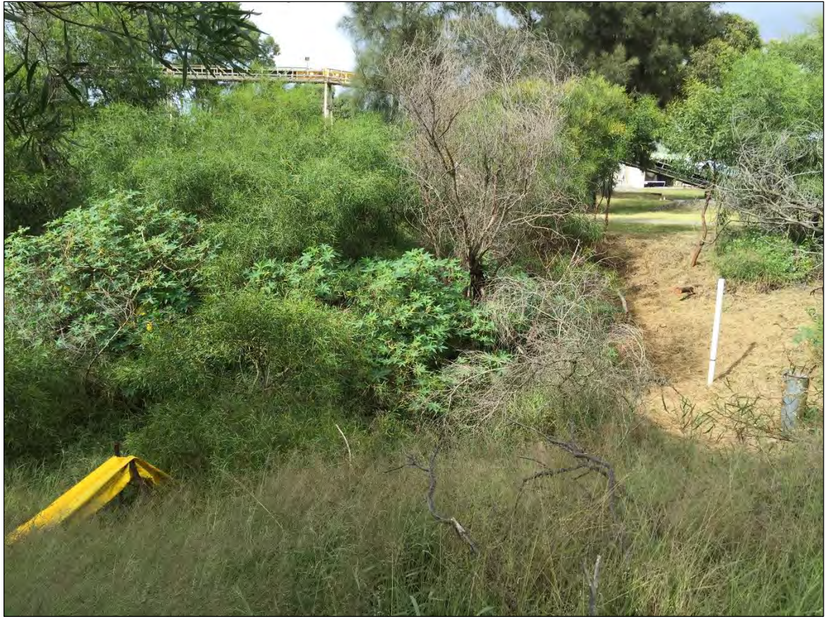
Plate 7 – The low (western) point of the constructed central drainage feature, with regulated storm water release valve on right and exotic Castor Oil plant along centre of drainage line.
