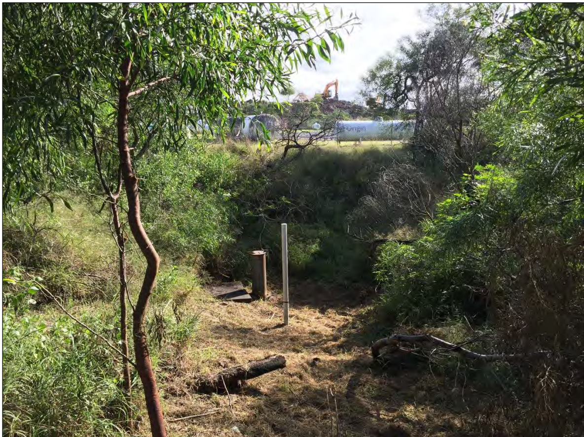
Plate 6– The low (western) point of the constructed central drainage feature, with regulated storm water release valve in centre of the plate.
