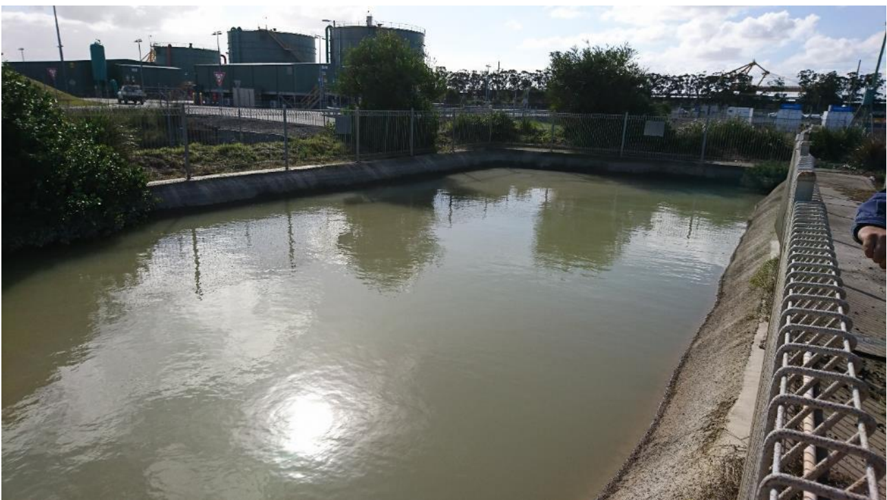
Photograph 3.2 The concrete basin
