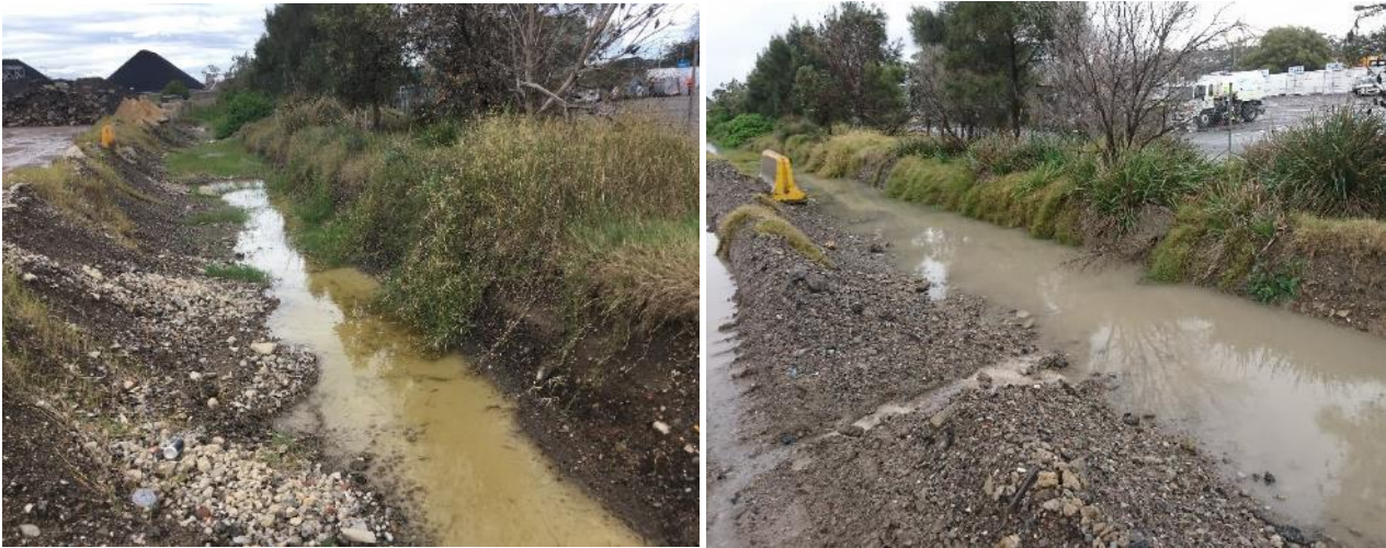
Photograph 3.1 Infiltration swale - the image on the left was taken in March 2019, after 50 to 60 mm of rainfall. Only minor amounts of surface water runoff occurred from this event. The image on the right was taken in August 2019 after approximately 80 mm of rain. Significant surface runoff from the yard occurred from this event.
