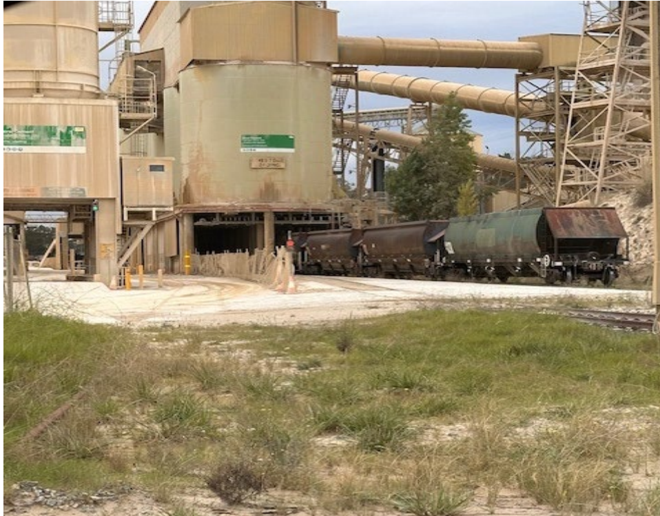
Train loading facility
