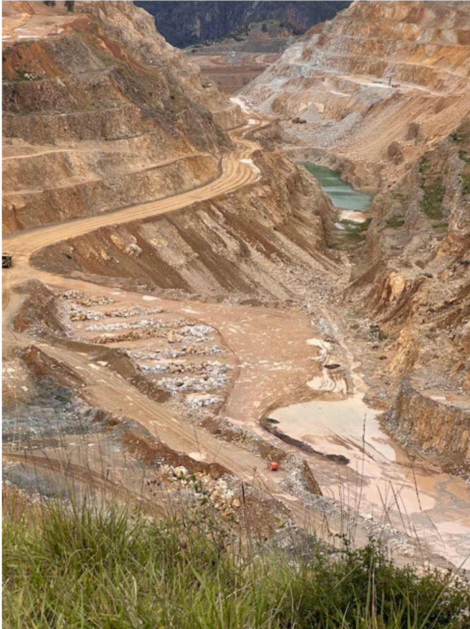
Mine water management, with laydown rows of limestone visible to drain into site water management system
