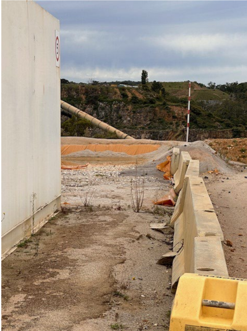
Bunded lining visible as orange sheet material
