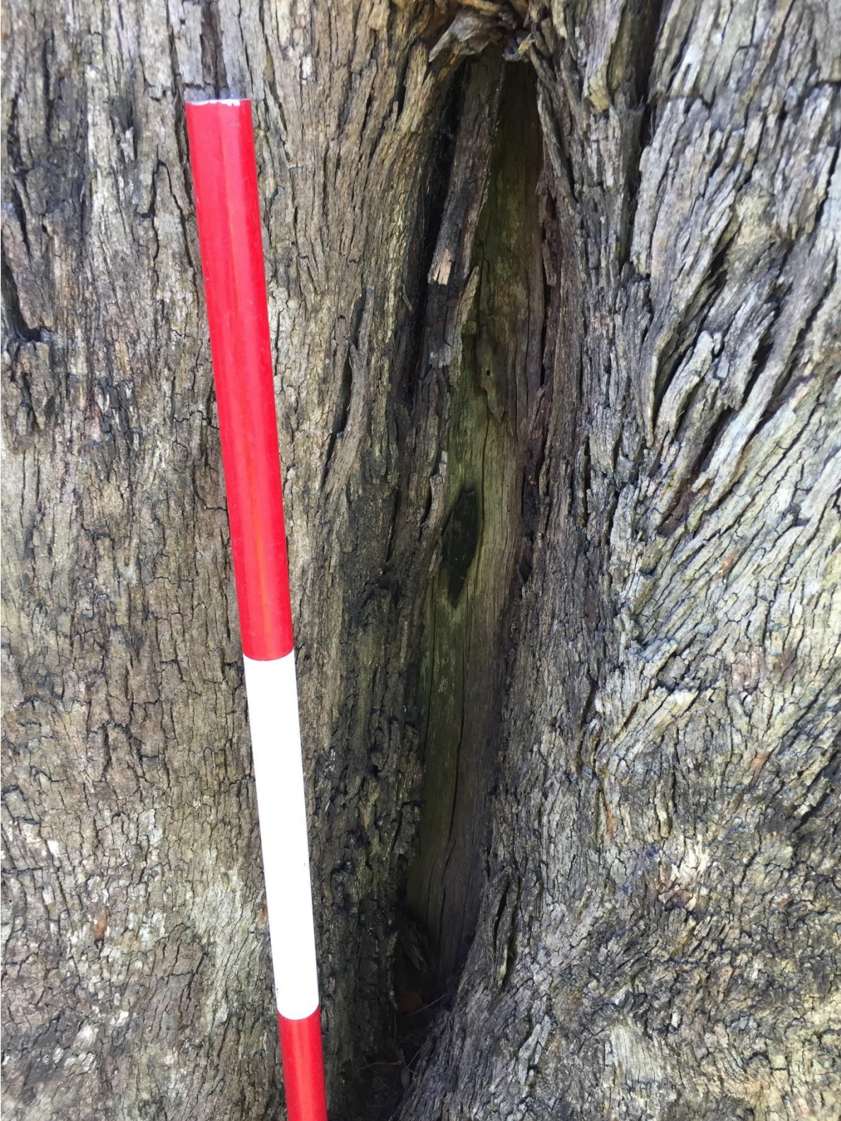
Photo 7: Close-up view of the Tree 2 scar, showing deeply overgrown margins and a narrow vestigial exposed dry face.
