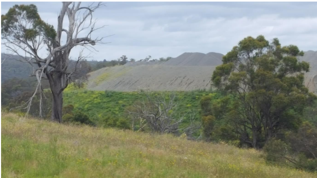
Plate 18 – Northern side of overburden emplacement showing first 10 m lift of the noise bund with completed rehabilitation. The second bench being unshaped scalps stockpile
