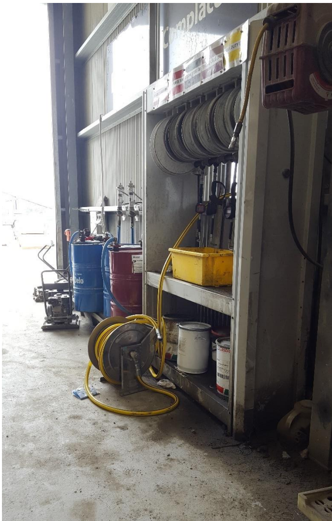
Plate 6 – Workshop Oil and Grease Dispensing hoses and reels
