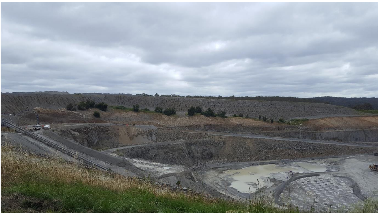
Plate 2 – Quarry Extraction Area showing drill pad prior to blast and unshaped overburden in background
