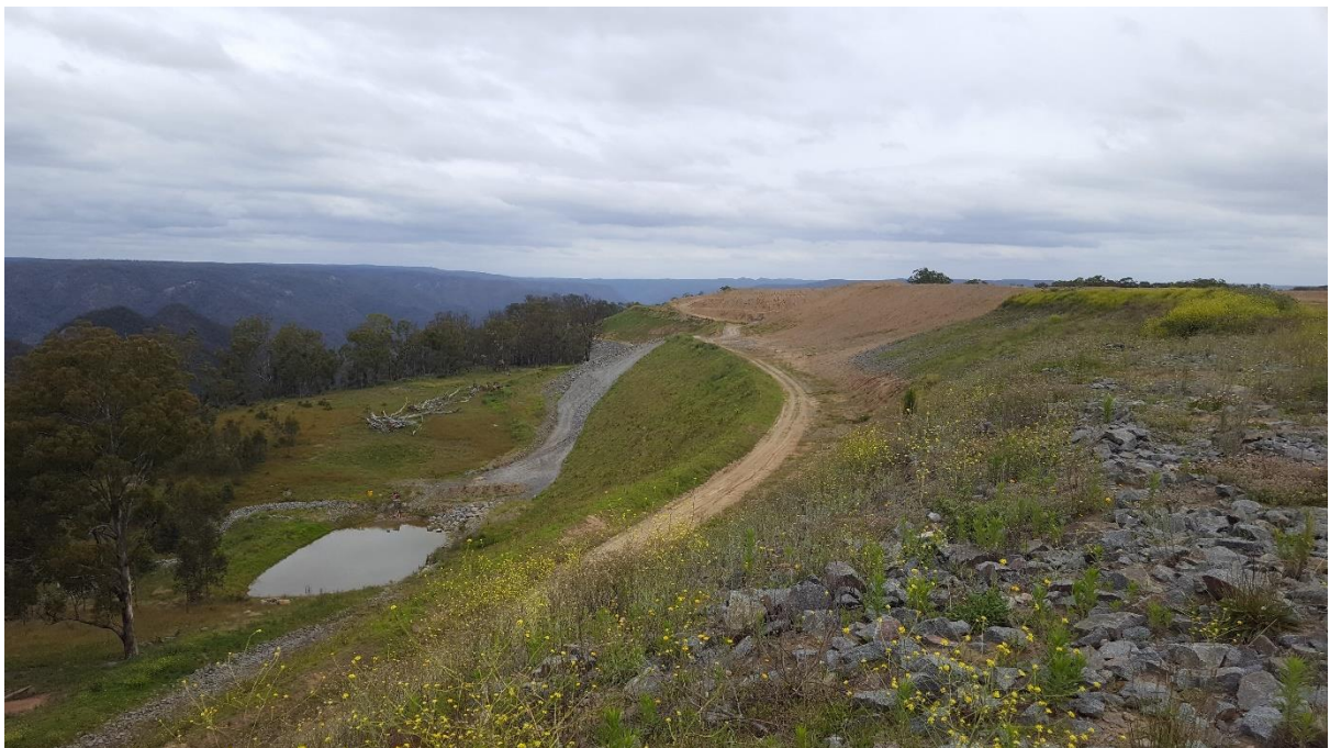
Plate 16 – Southern Face of Overburden Emplacement showing progressive rehabilitation, benching and sediment ponds
