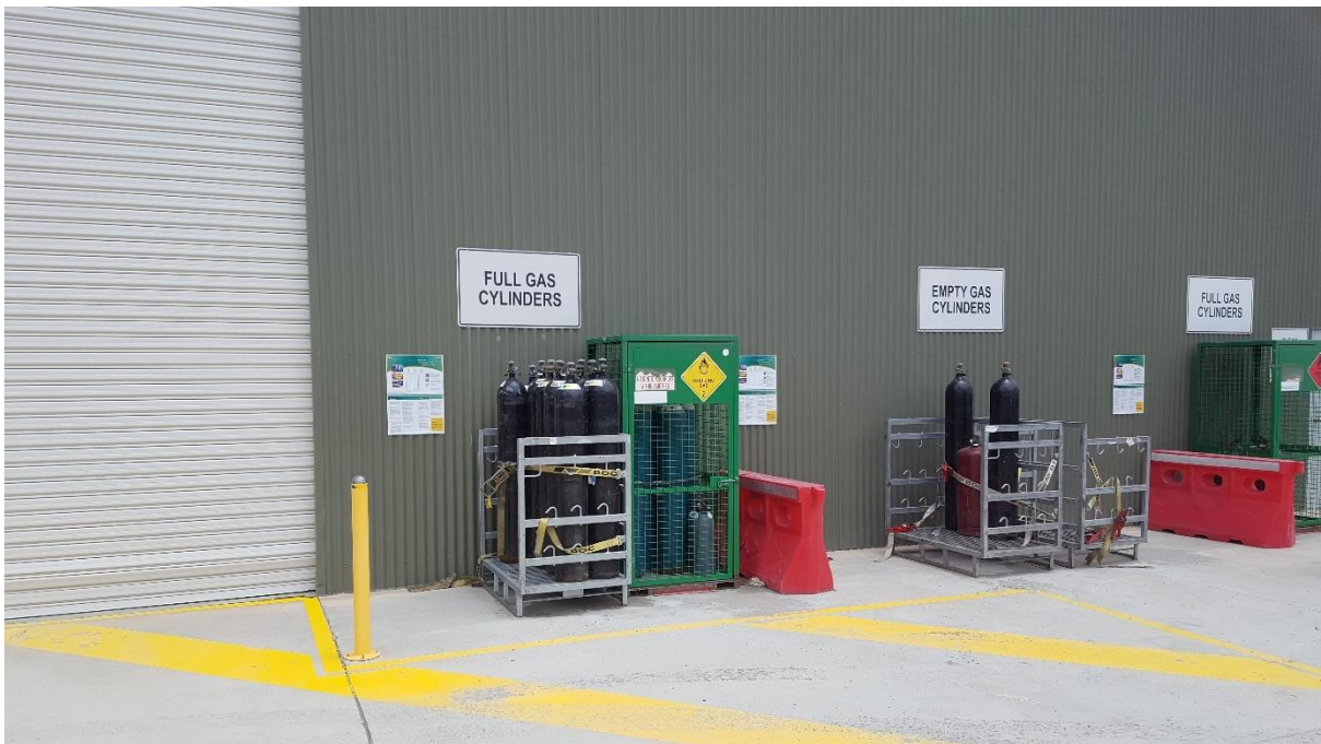
Plate 8 – External Wall of Workshop showing separation of Acetylene and Oxygen cylinders
