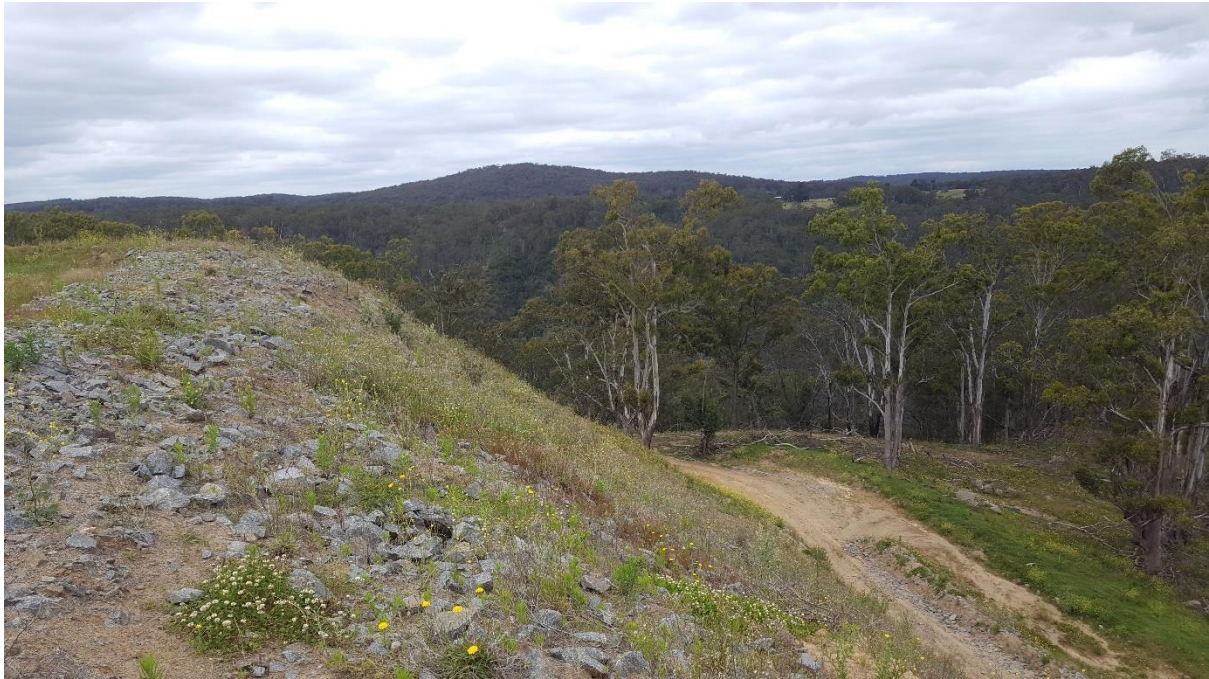
Plate 17 – Rock Armoured section of outer emplacement wall
