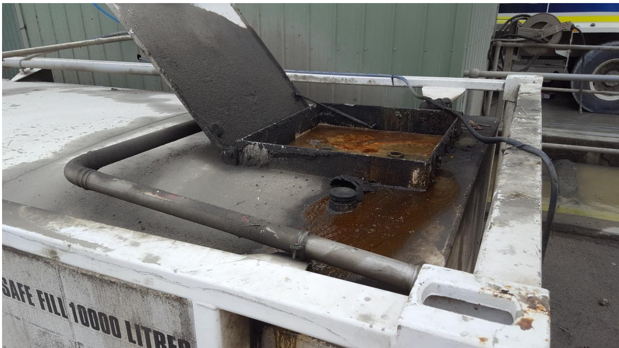
Plate 4 – Inspection of Waste Oil Tank
