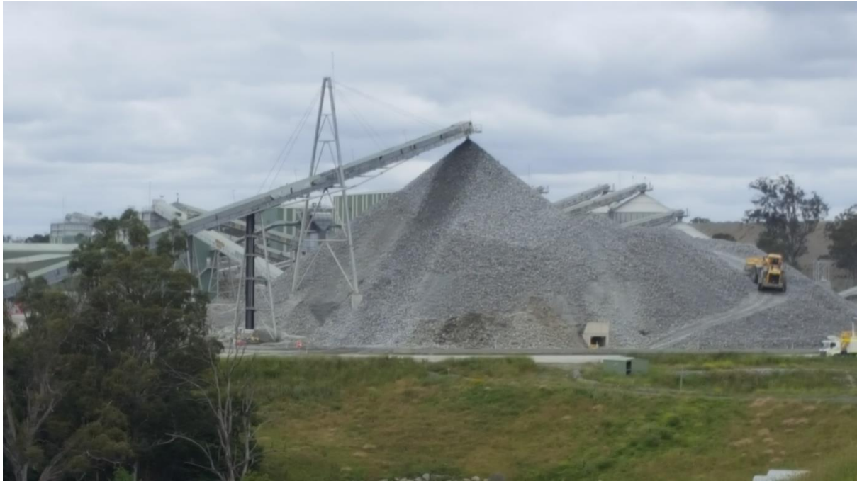
Plate 11 – Primary Crushed Rock Stockpile prior to entering secondary processing plant
