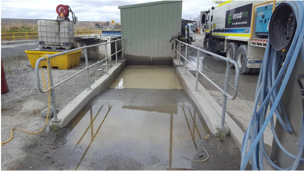
Plate 5 – Washdown Bay and silt sump
