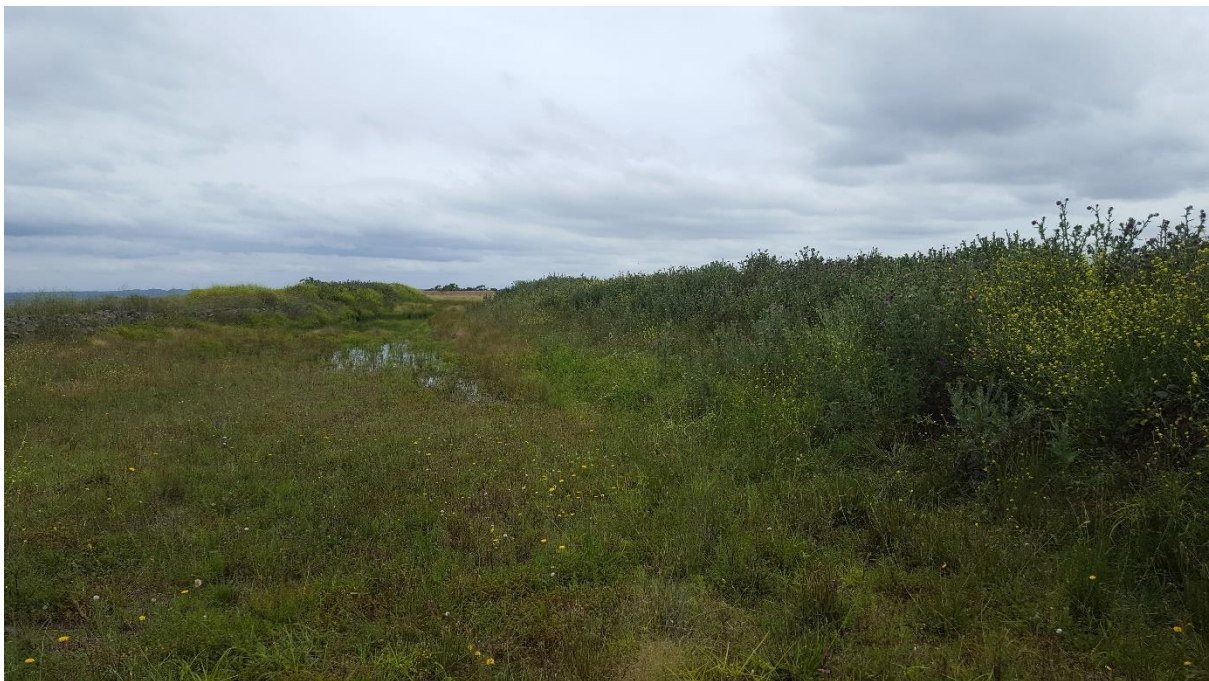
Plate 14 – Top of Overburden Emplacement showing progressive rehabilitation
