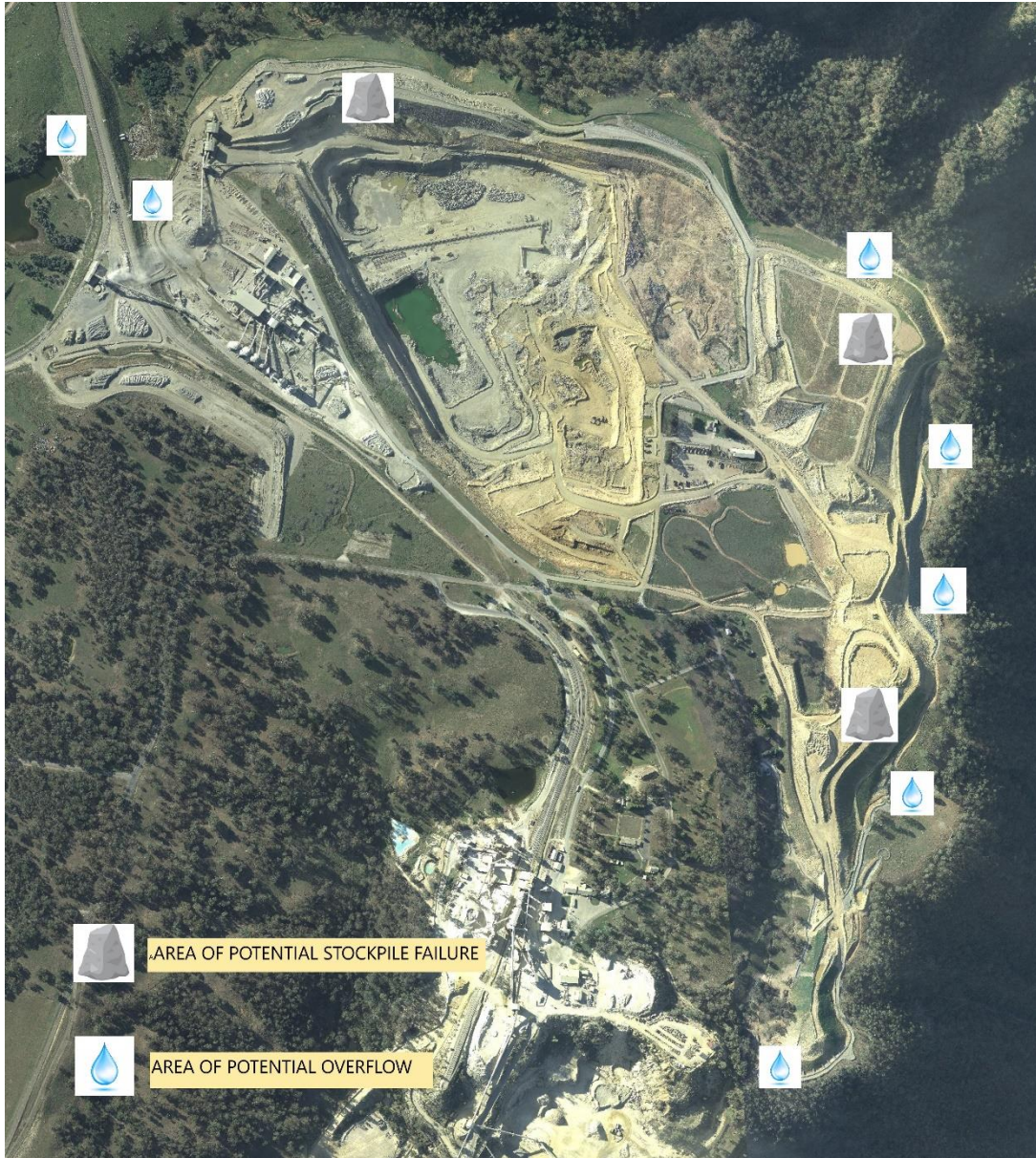
Figure 4: Overflow of Sediment Dams due to Flooding or Dam Failure
