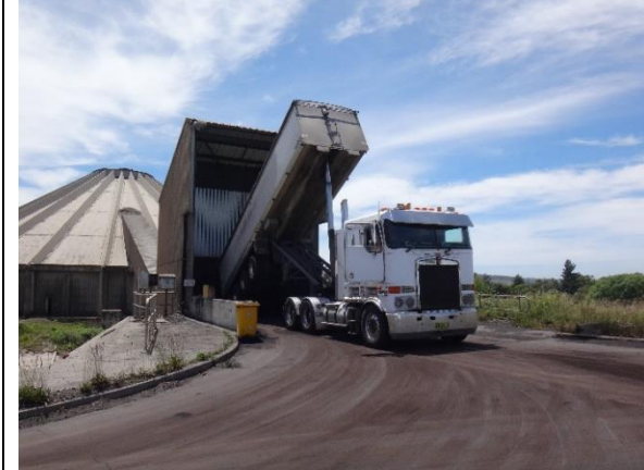
Photo 9- Truck dumping coal into hopper
