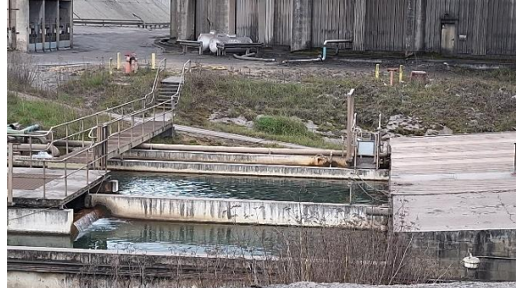
Photo 10 - Water Treatment Ponds
