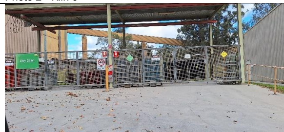
Photo 4 – Oxy-Acetylene Storage
