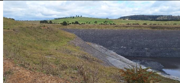
Photo 18 – Shale Quarry Rehabilitated Batters
