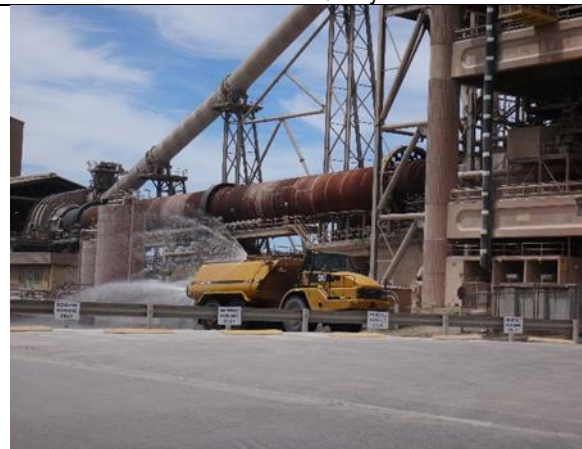
Photo 22- Water cart used for dust suppression
