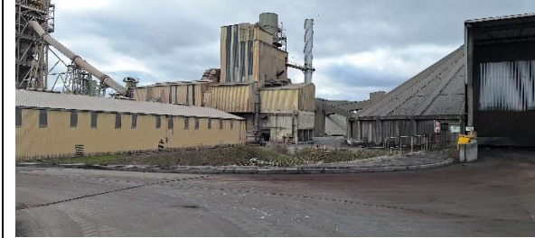
Photo 7 - Coal Reveal and Furnace
