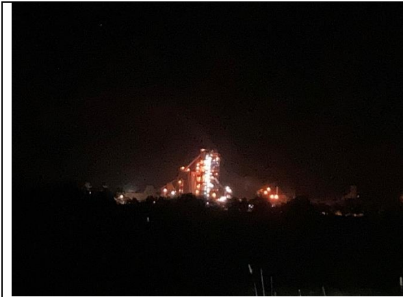
Photo 31 – Plant from Berrim Road
