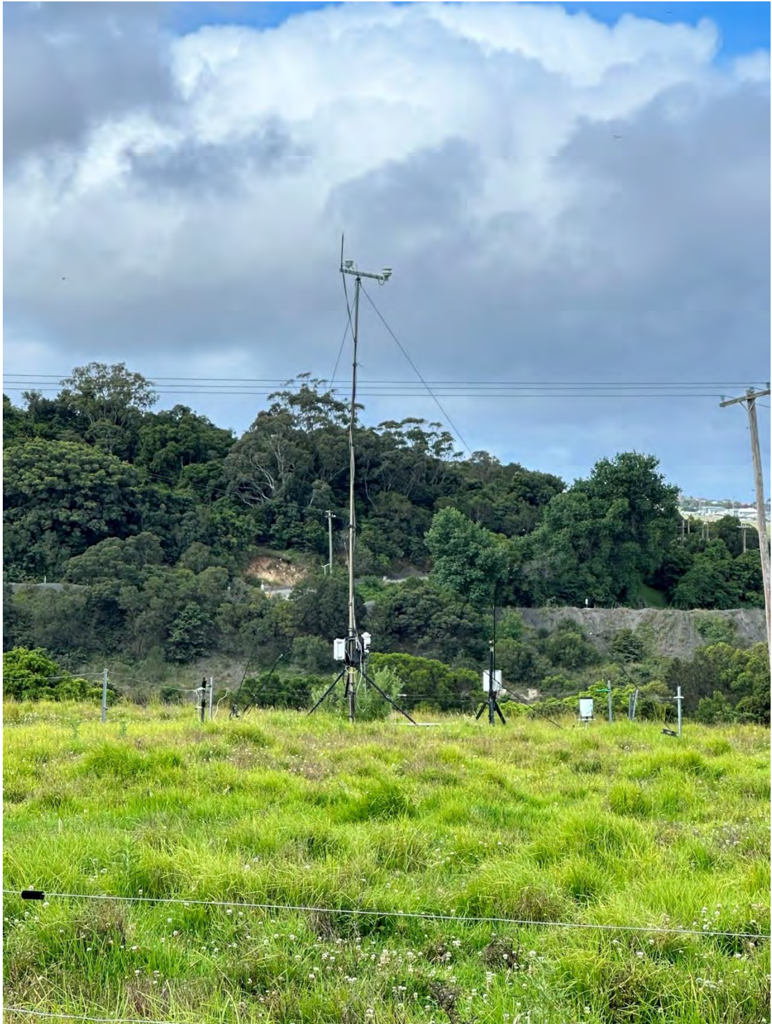
Example of offsite weather station and air quality monitoring equipment.
