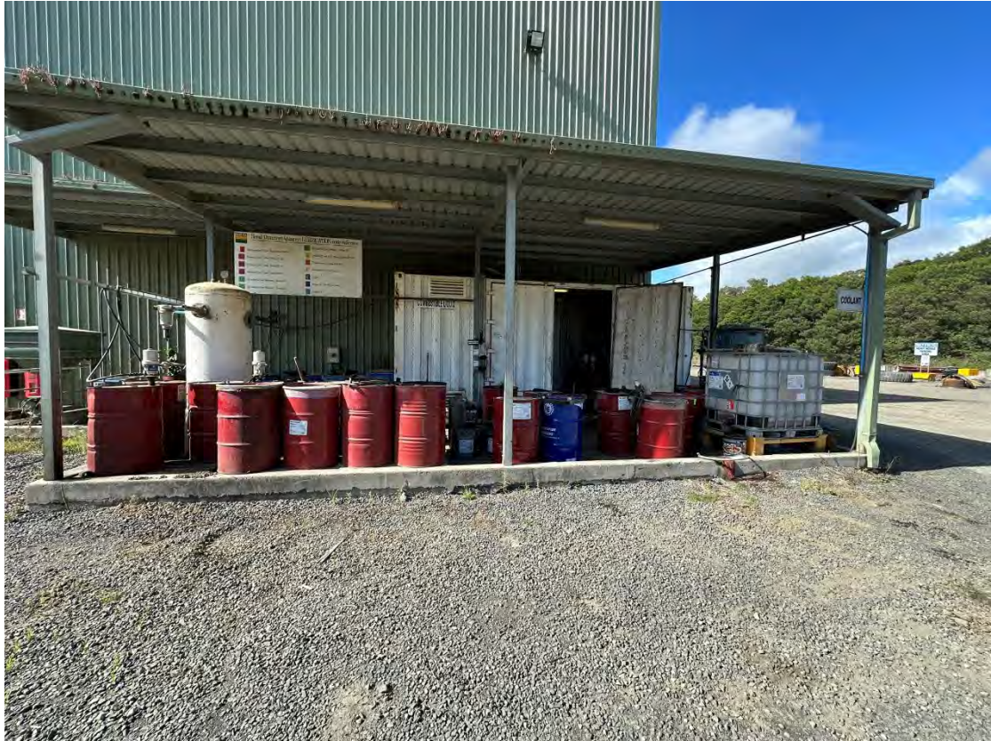
Oil drums being correctly stored in bunded area near maintenance workshop.
