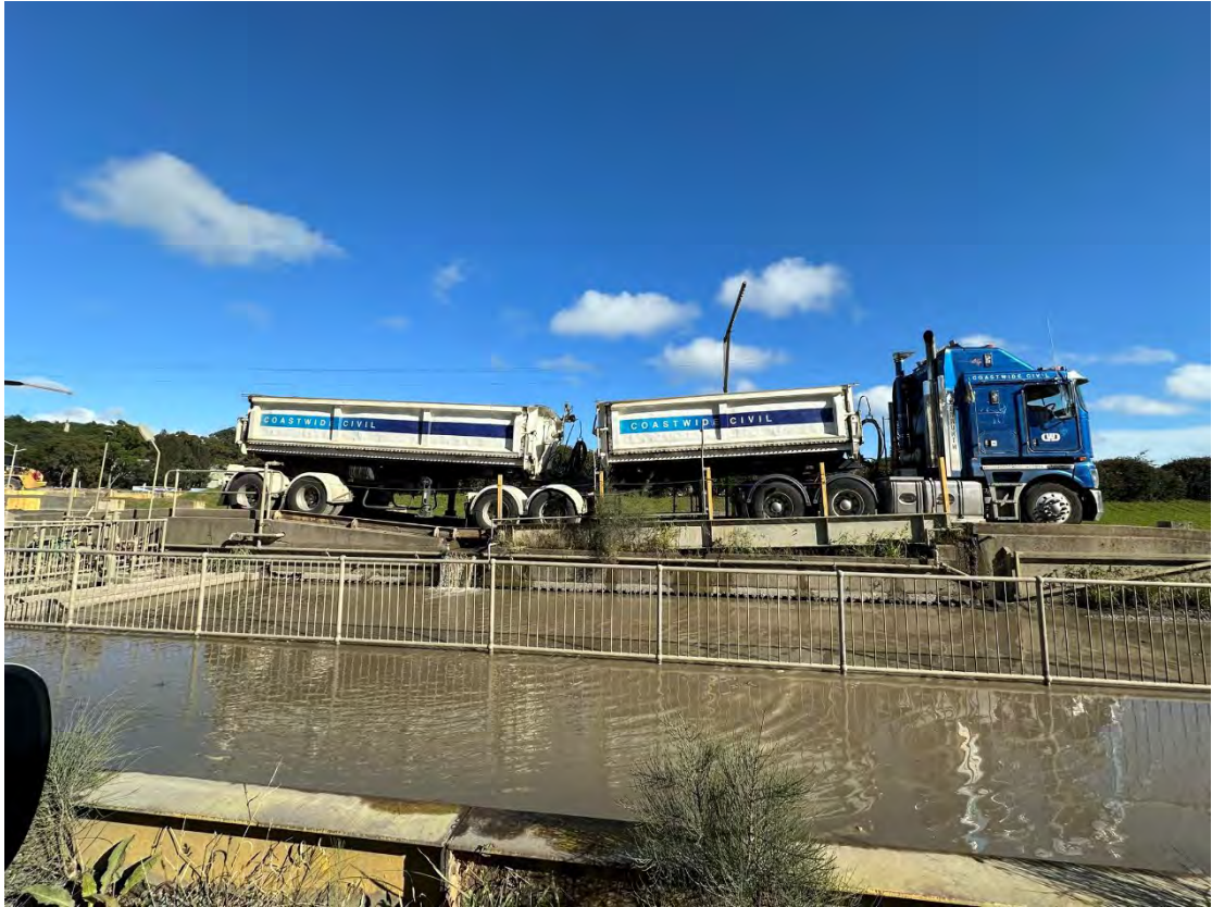
Example of truck using wheel wash.
