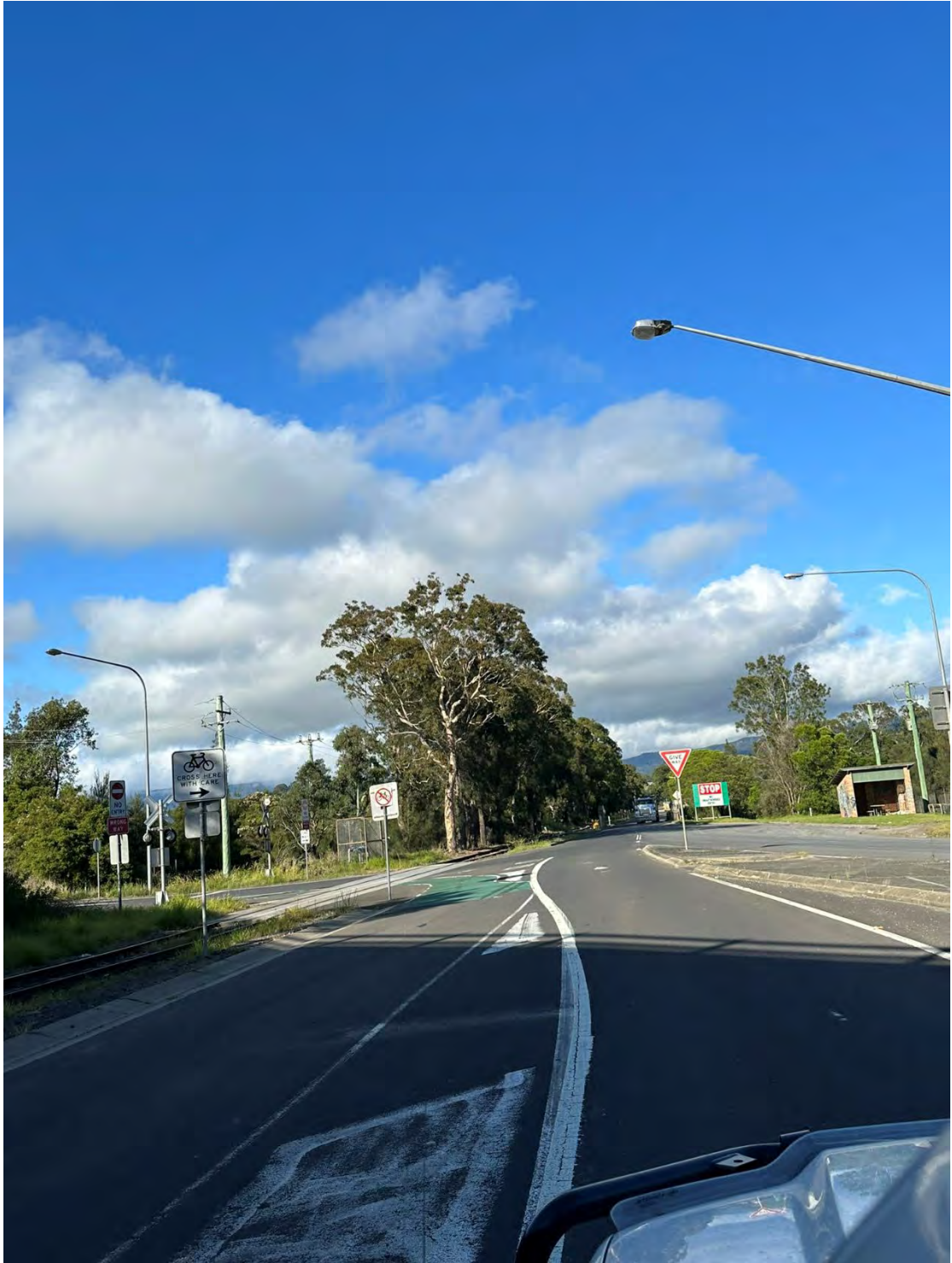
Entry and exit at Tabbita Road.
