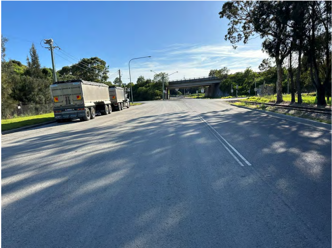
Clean entry and exit conditions at Tabbita Road.
