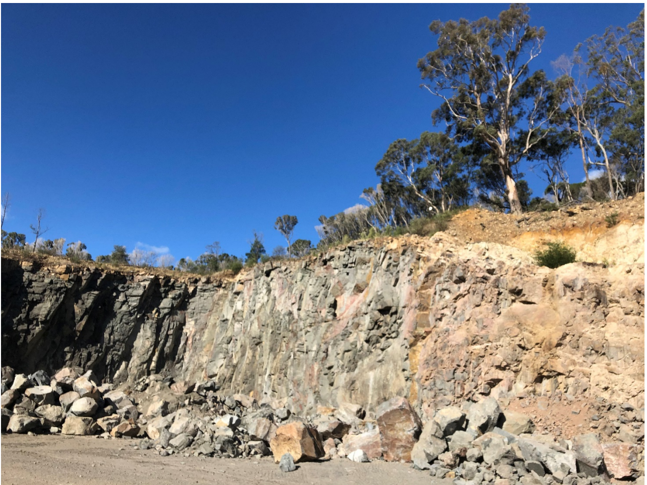
Photograph 3.2 Looking at the South Croome Ramp area undergoing blasting and removal
