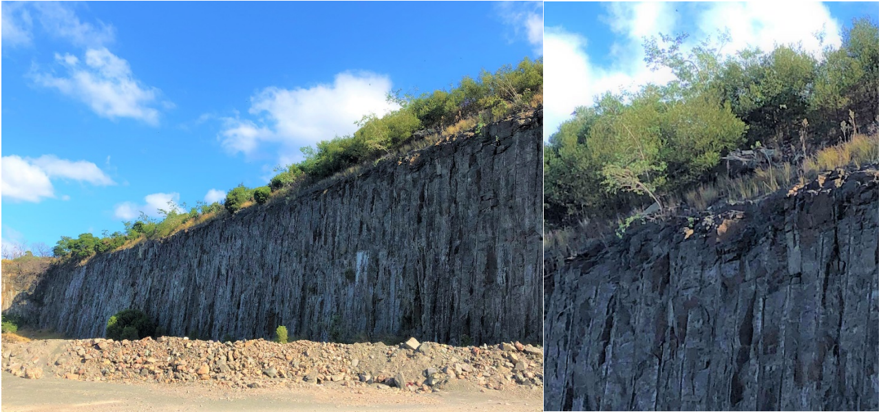
Photograph 3.1. Looking at Rehabilitation area located in South Croome
