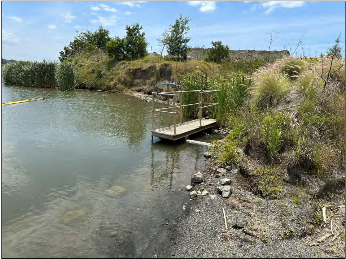
Stage 2 water release valve location
