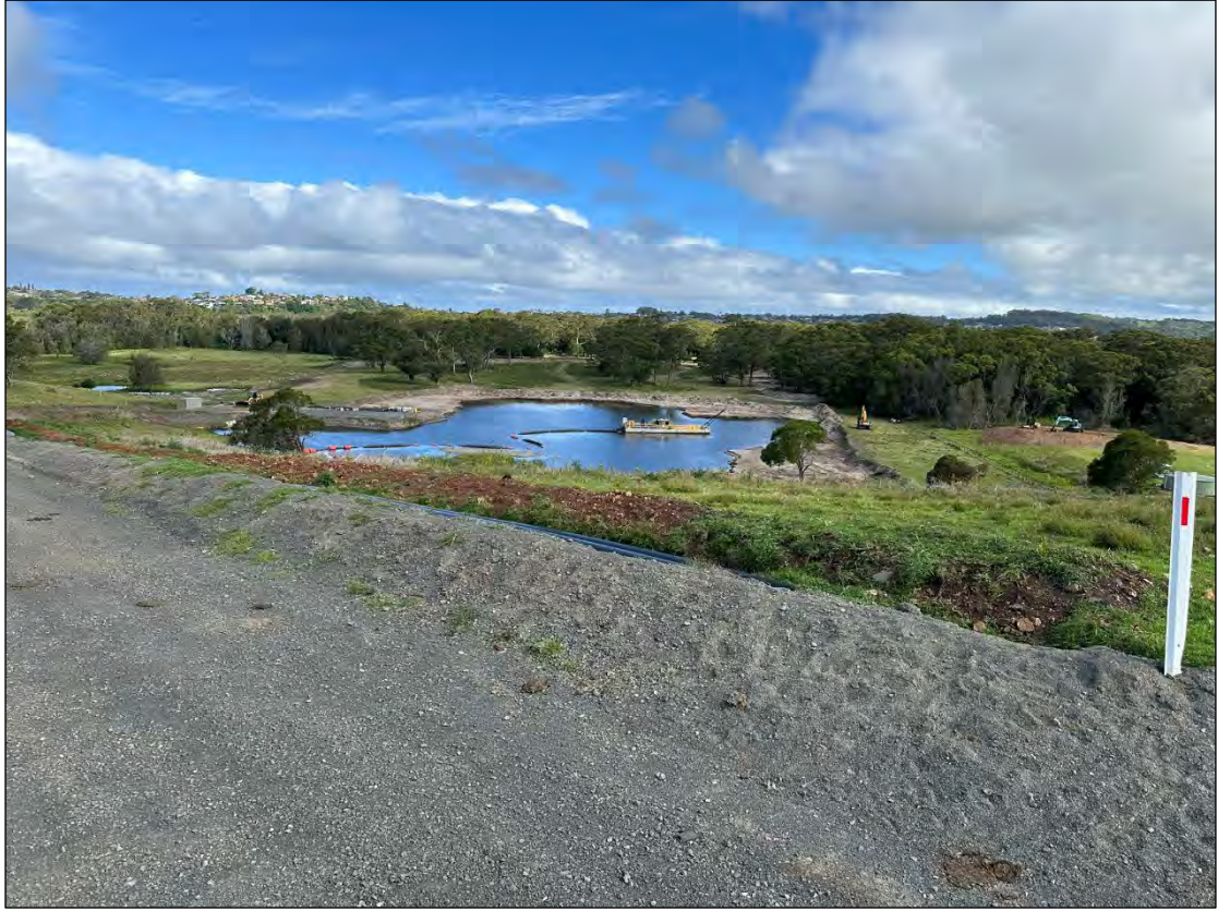
Stage 5B active extraction area
