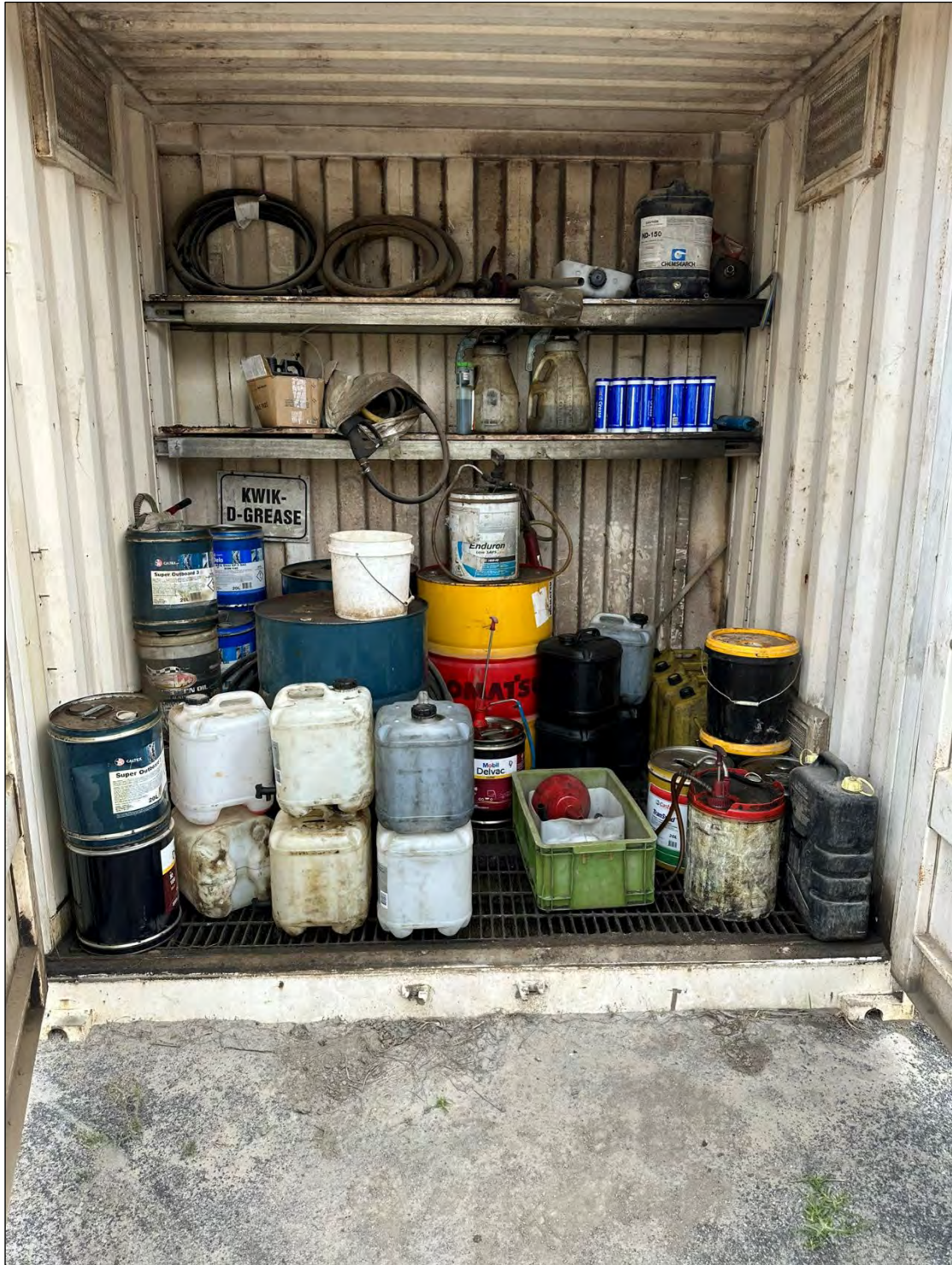
Grease and oils storage with bunding
