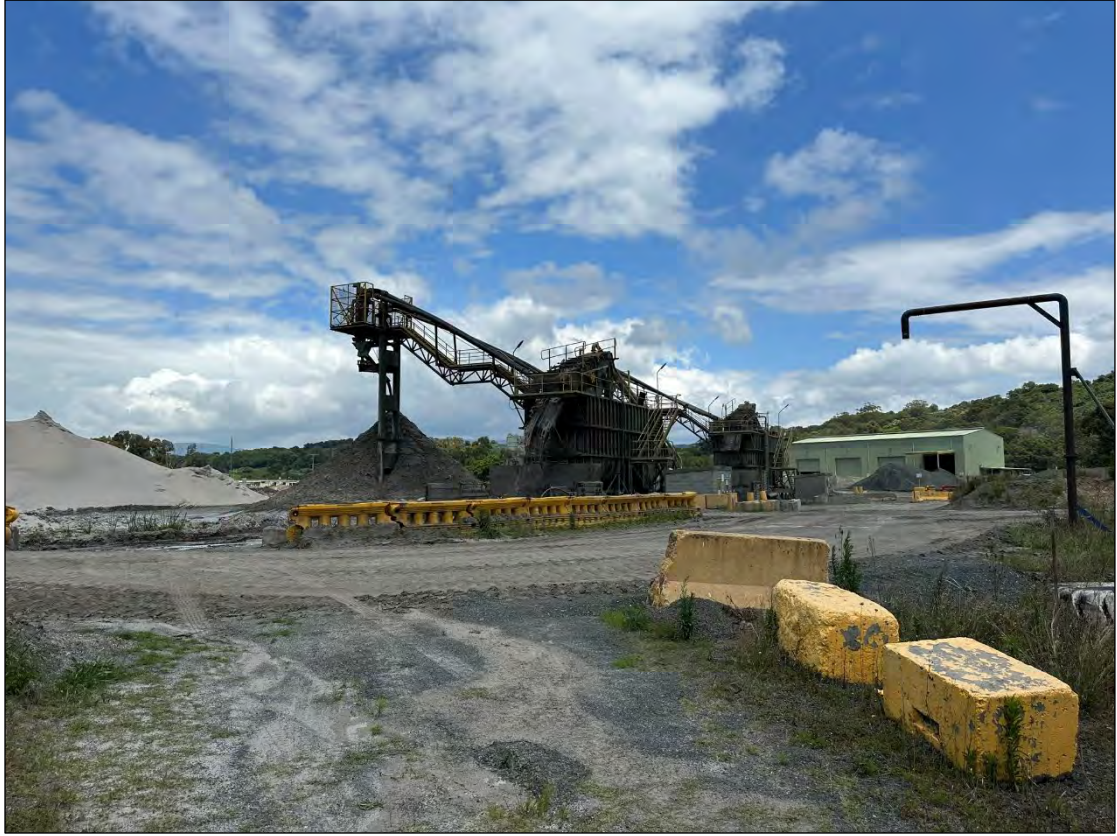
Sand and water separation plus storage area with workshop in background
