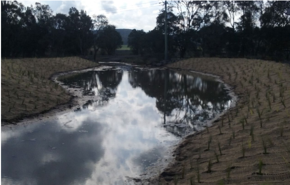
FY17 Re-aligned Western Tributary Rehabilitation Progress
