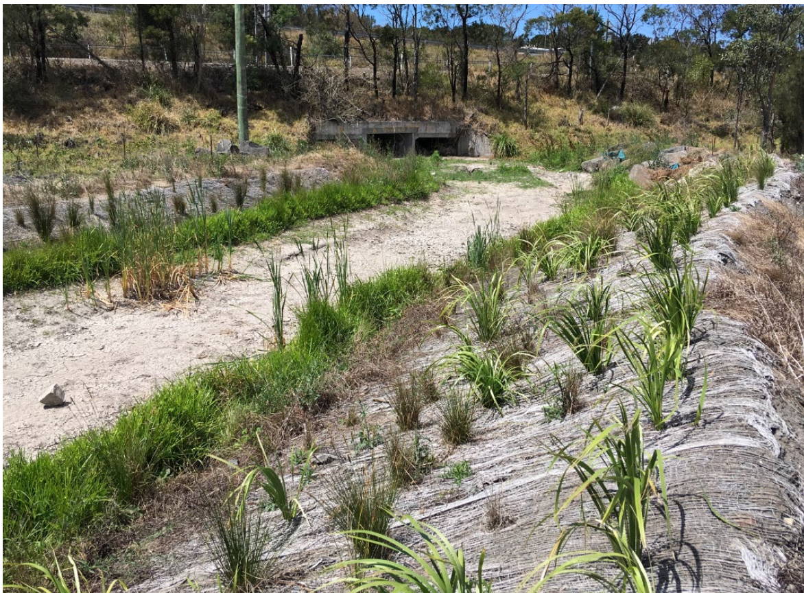
FY18 Re-aligned Western Tributary Rehabilitation Progress
