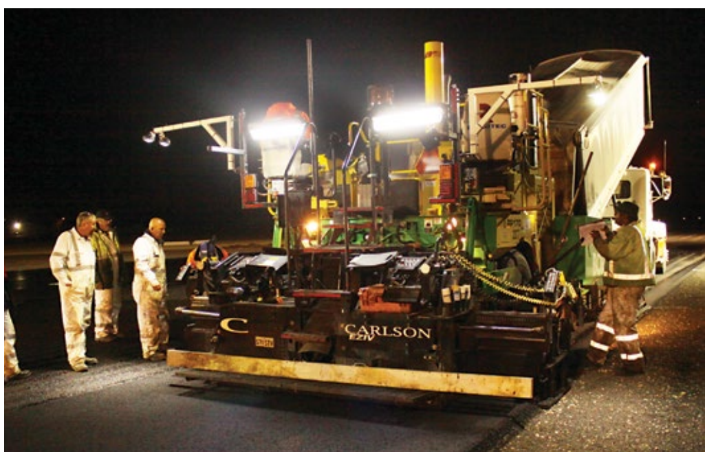
Asphalt crews work to build tarmac each night.
