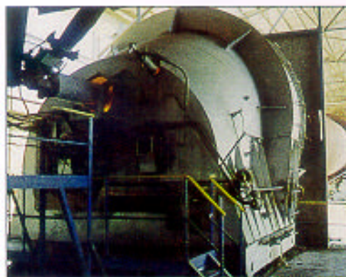
BCSC Rotary Kiln at Warrn Ponds
