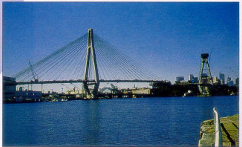
The Glebe Island Bridge, Sydney
